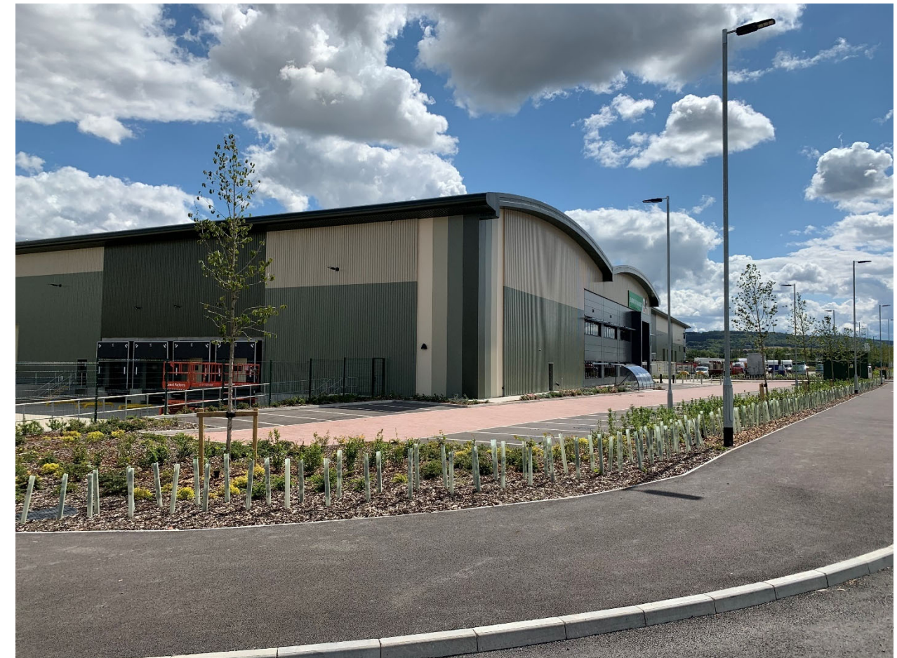
Fig 49. Column mounted and building mounted, light fittings for the development plots and highways.
