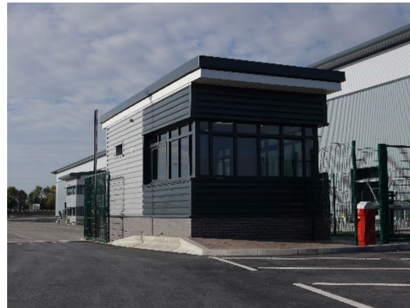
Fig 50. Example of gatehouse at entrance to service areas.
